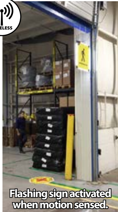
Sign is dormant if no motion in sensing field.
