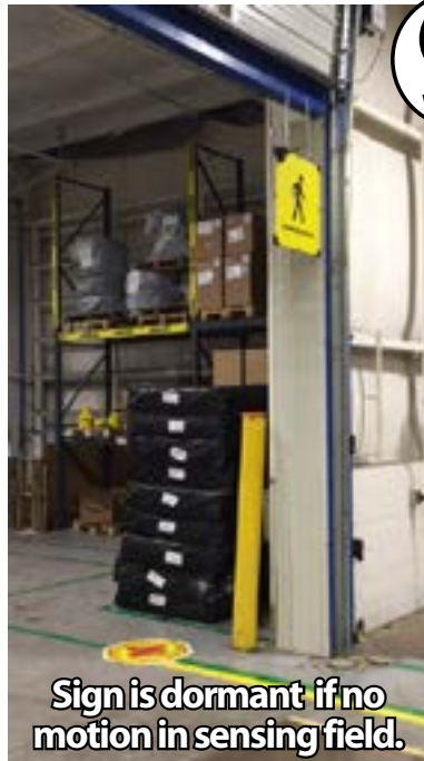
Flashing sign activated when motion sensed.
